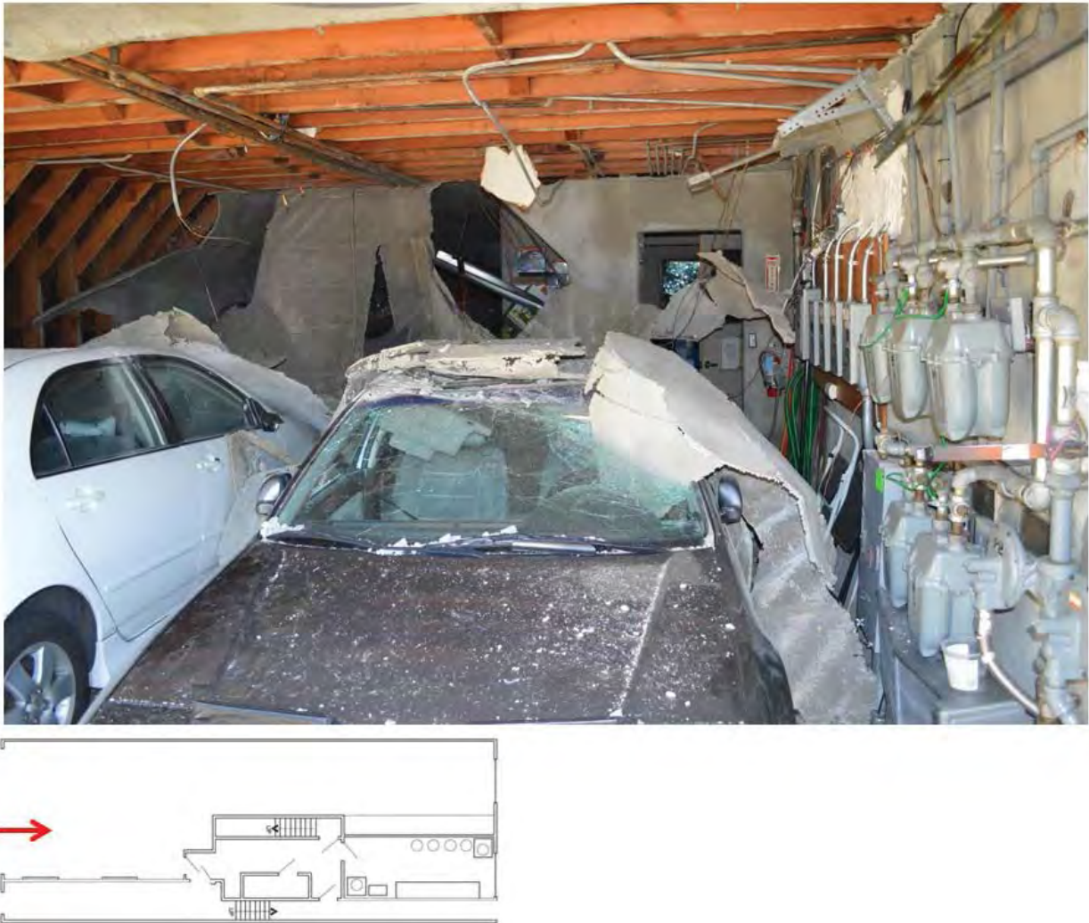
Figure 7. Front of garage at incident house. Photo taken by Exponent on November 27, 2017.
