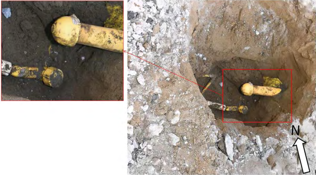
Figure 27. End cap on west end of abandoned 2-inch plastic service line.
