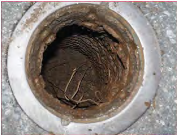
Figure 20. Unmapped valve on cross-tie. Square valve operator faintly visible in the mud. Photos taken by Exponent on November 27, 2017.
