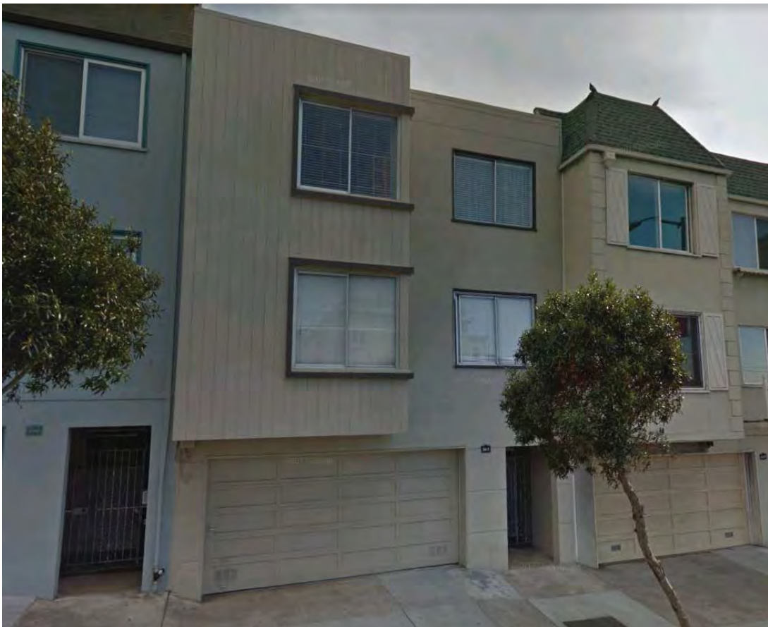
Figure 2. [REDACTED] prior to incident. Image from Google Maps. Image date: November 2016.
