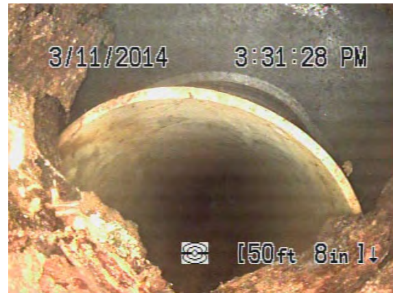
Figure 6. Offset joint 50 ft. from entry on property
