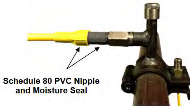
Figure 4. Installation of Schedule 80 PVC Nipple
