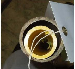
Figure 7: 1-1/4 plastic main inserted into 2 inch steel.
