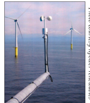
A Campbell Scientific system monitors an offshore wind farm in North Wales.
