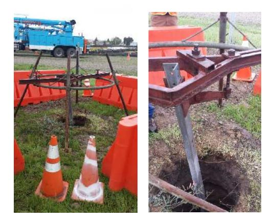
Figure 6 – Sample of a template ring holding a foundation stub
