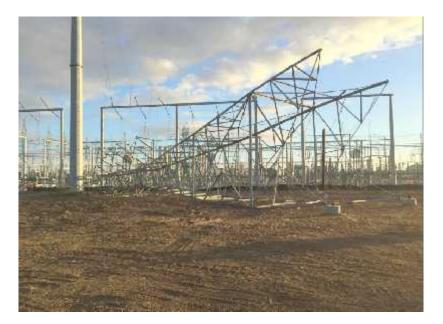
Figure 11 – Collapsed Tower 61/268
