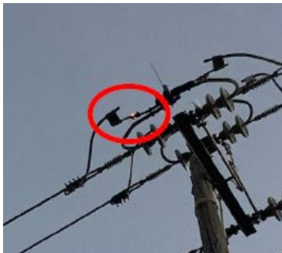
Figure 3: Glowing bolt and switch equipment from 20 Day Report.
