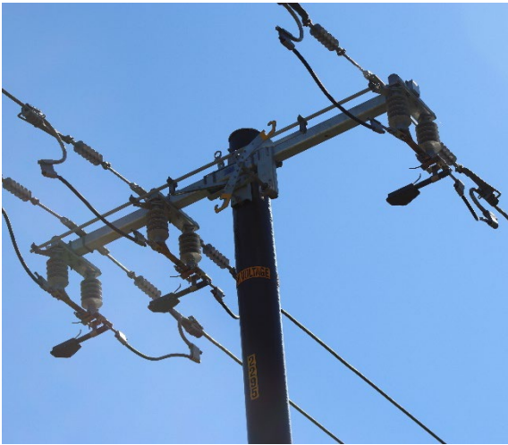
Figure 5: New equipment on top of pole.
