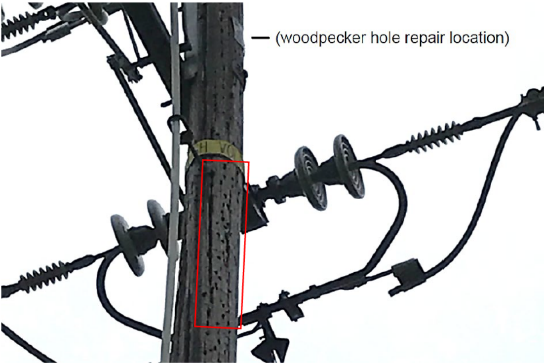
Figure 12: Incident Pole with repair of the single large woodpecker hole indicated and showing the excessive woodpecker damage which was noted after that repair.
