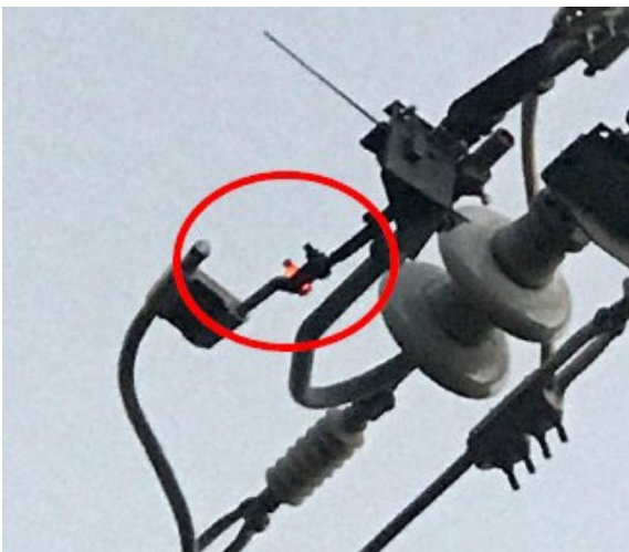
Figure 2: Glowing bolt identified in 20 Day Report.
