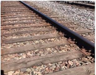
Track section with loose and missing fasteners
