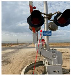
Gate arm light wire can easily become entangled on light housing preventing the gate from moving down when crossing is activated
