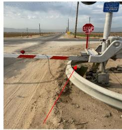
Gate arm light wire can easily become entangled on the barrior preventing the gate from moving up after train leaves the crossing
